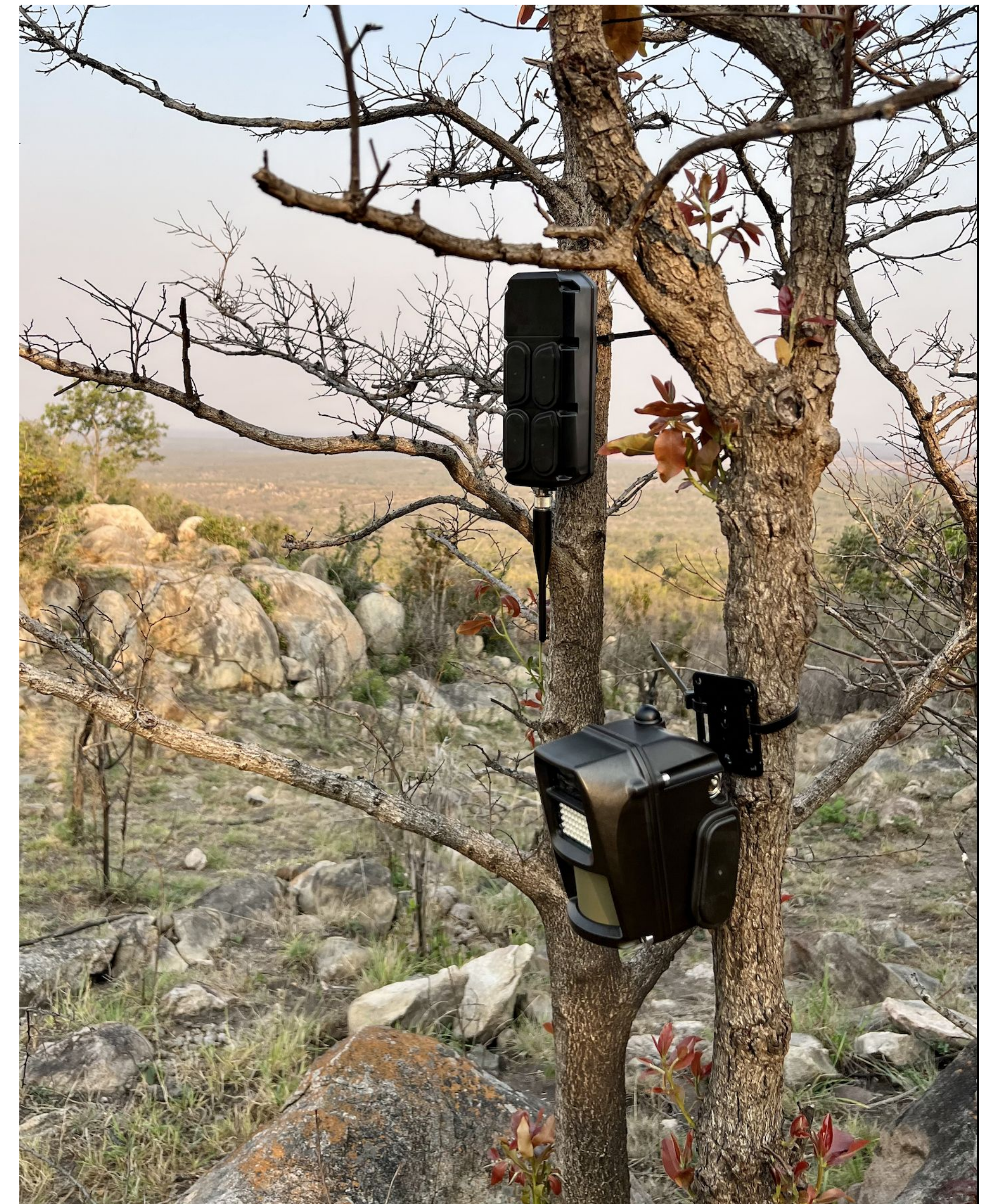
installed Reconeyez system: Bridge & Detector
